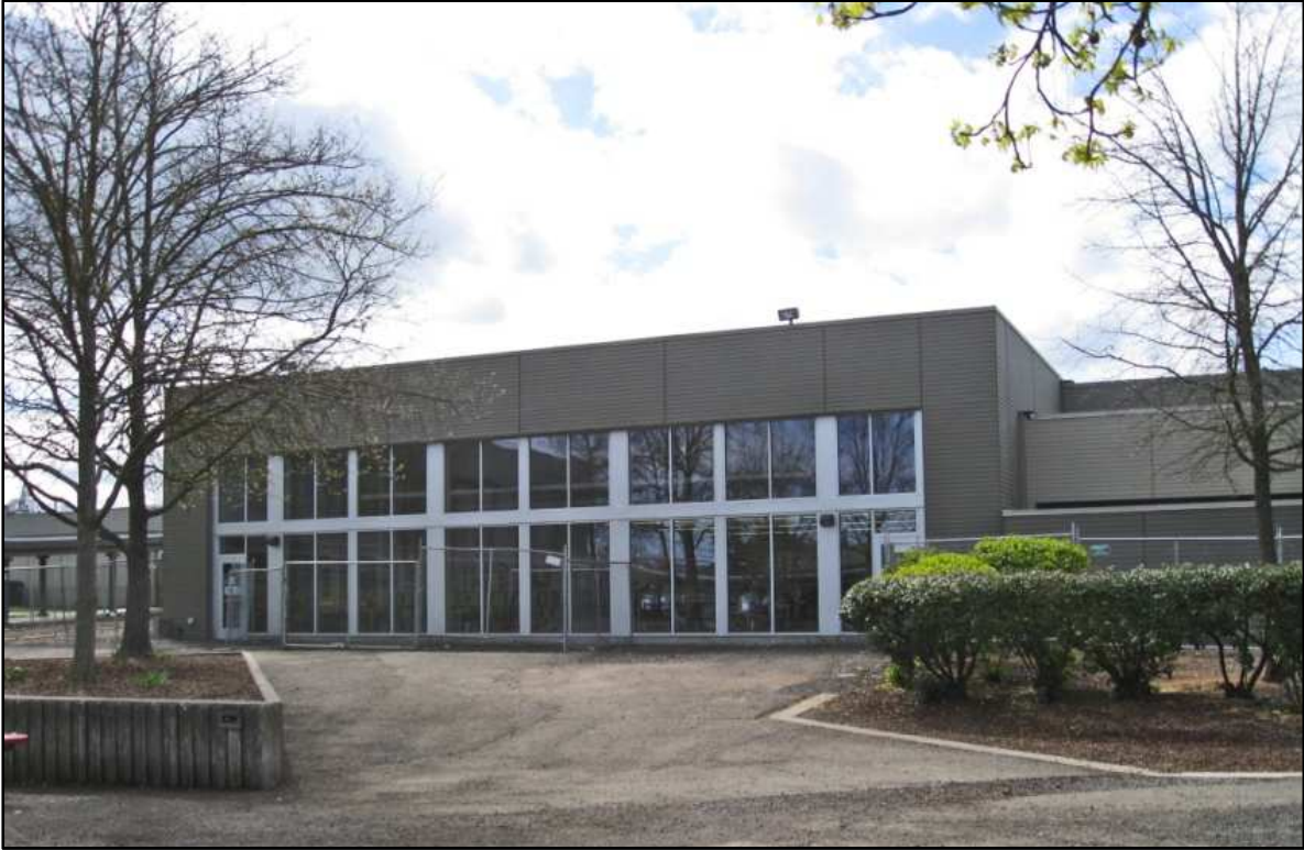
Media Center Exterior – North Elevation
