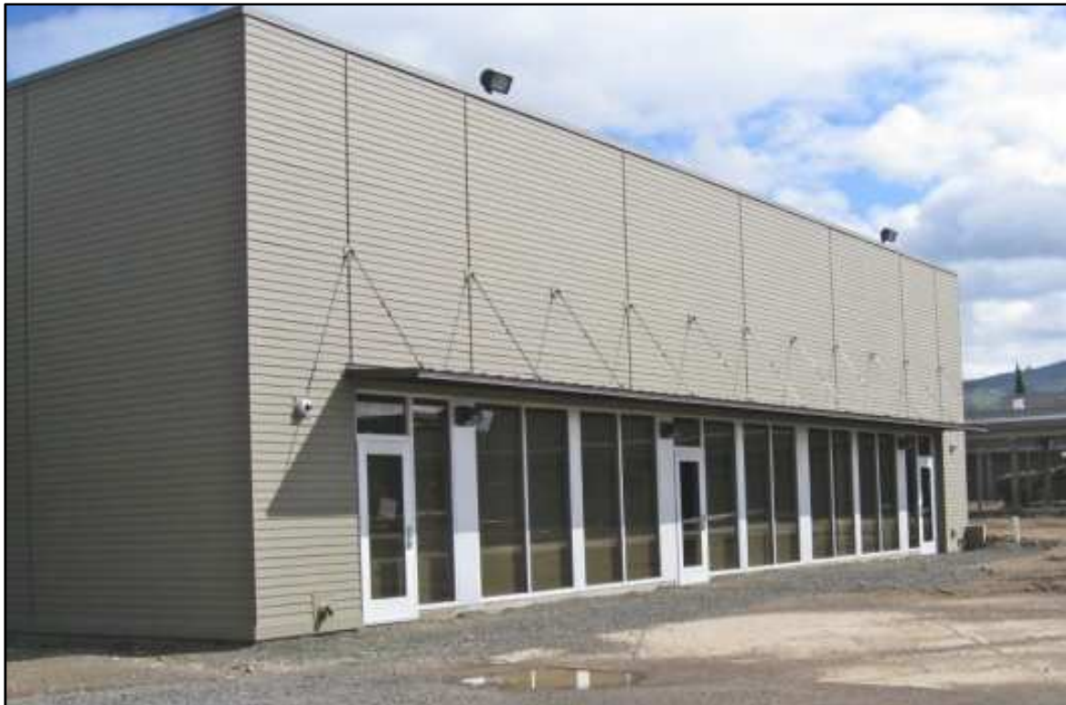
Classrooms – South Elevation
